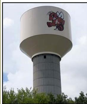
Completion of the Dyche Lane elevated water storage tank construction is drawing near. This project involved the design and construction of a 500,000 gallon composite water storage tank that replaced the existing metal tank. The tank will provide adequate water pressure and supply to a large part of the City and has an estimated useful life of 20-25 years.
